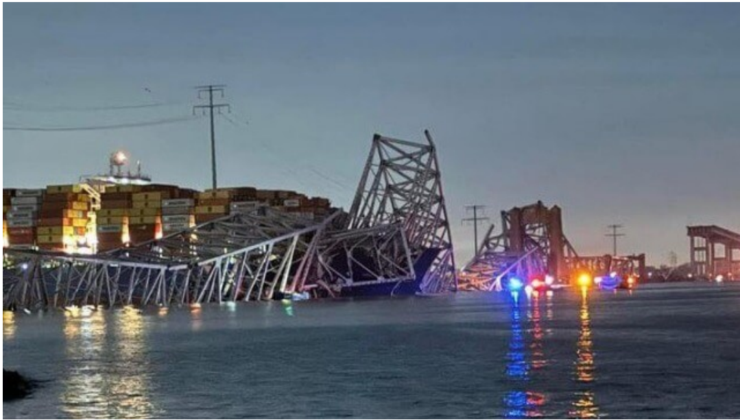
Baltimore's main road bridge collapsed after a containership with one of the pillars (Harford Co., MD Fire & EMS)
