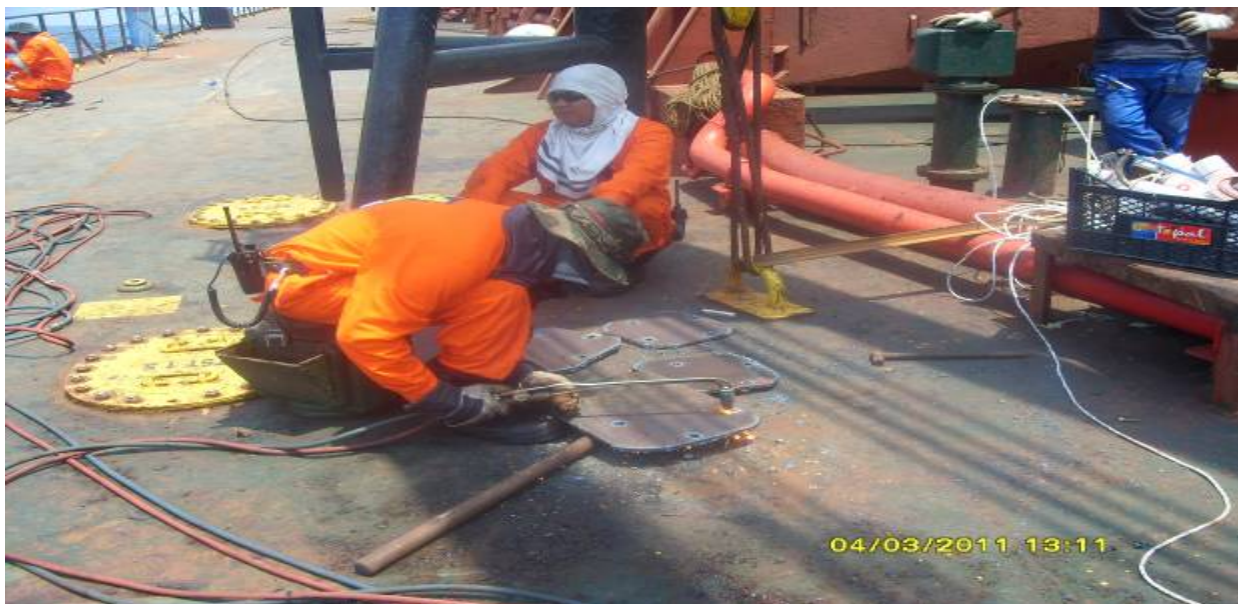
Photo no.9: 3 April 2011, salvage team taking preventive measures against flooding
